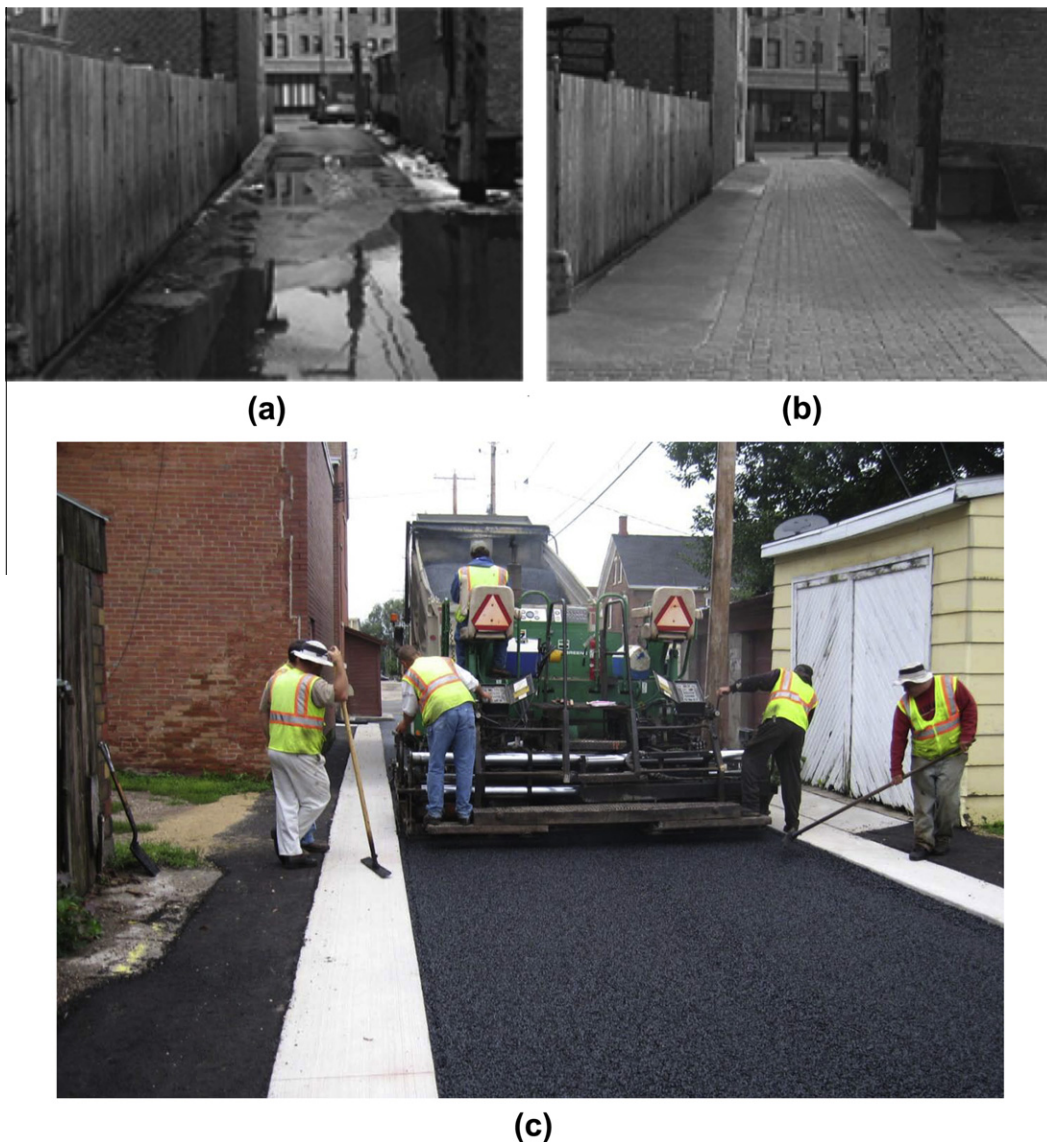
Fig. 1. Stormwater management retrofits in US alleyways. (a) A flooded, impermeably paved alley in Chicago. (b) The alley was resurfaced with permeable pavement. Source: Photo courtesy of the Chicago Department of Transportation (2010). (c) Dubuque's first green alley, being paved with permeable asphalt. Source: Photo courtesy of J. Dienst (2009).
